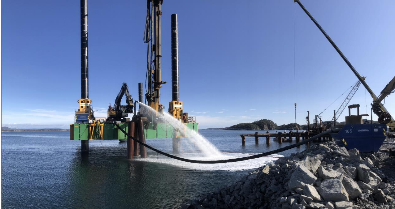
83.347 Cleaning of pile foot
